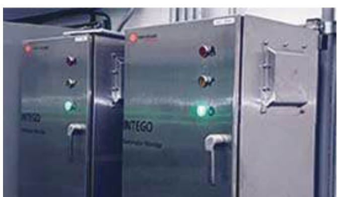
Intego For Generator Partial Discharge Monitoring
