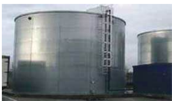
Fire Water Tanks
