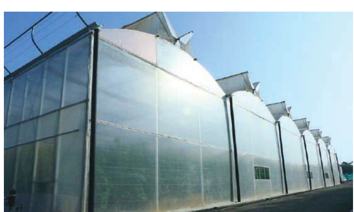
Greenhouse - Polycarbonate Sheet
