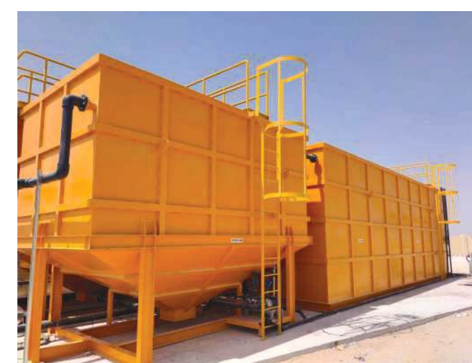
Sewage Treatment Plant
