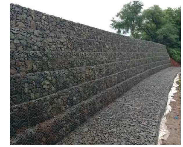
Gabion Mesh & Mattress
