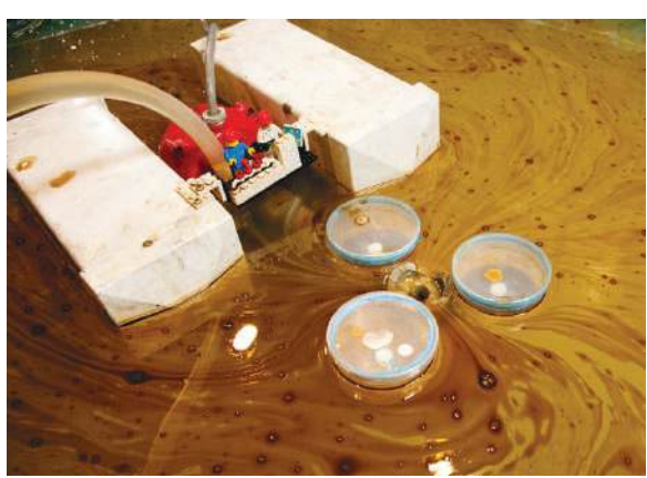
Oil Skimmer (Fog & Scum Removal)
