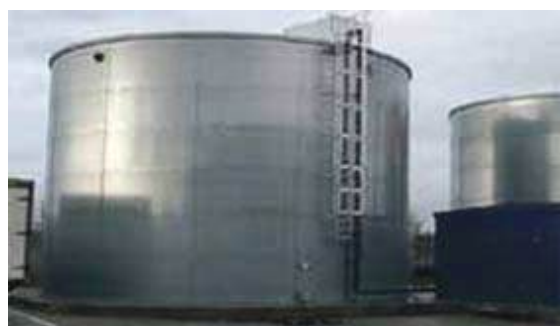
Fire & Potable Water Tanks
